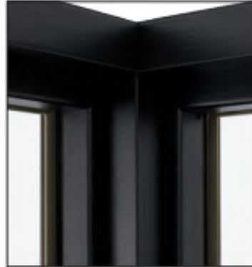
Interior Close Up
